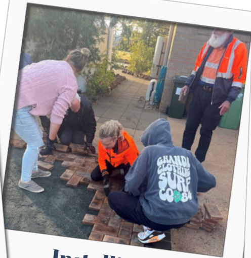
Installing a firepit @ WNLC
